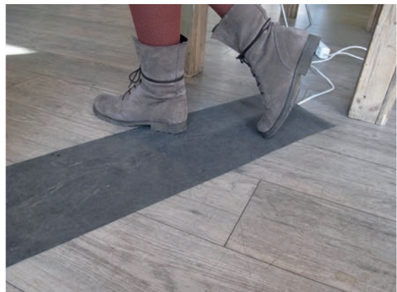
Safe: extension cords covered with rubber mats
